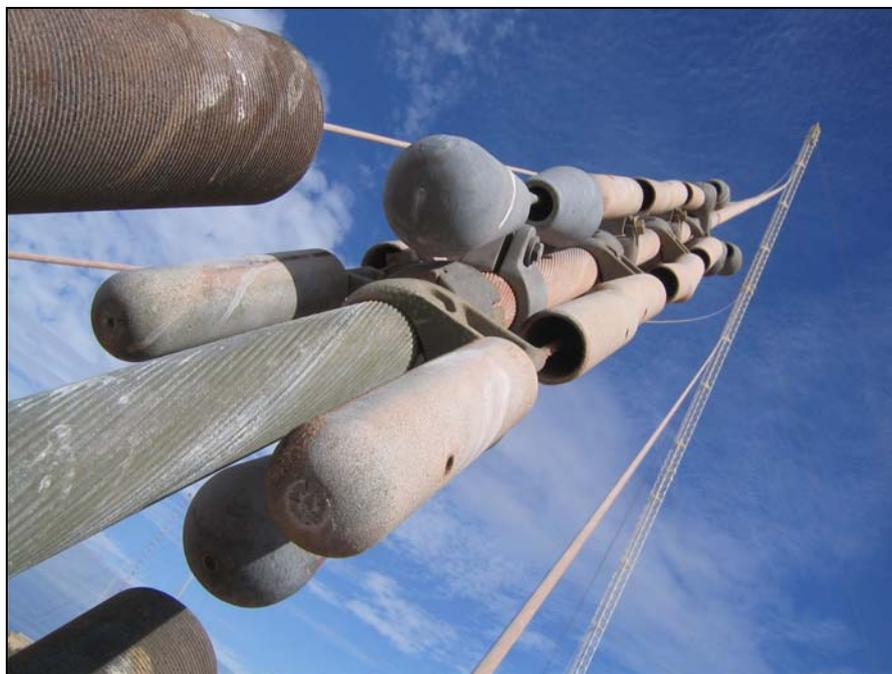
**FIGURE 1 - Typical guy supporting slender tower with vibration dampers at lower end**
